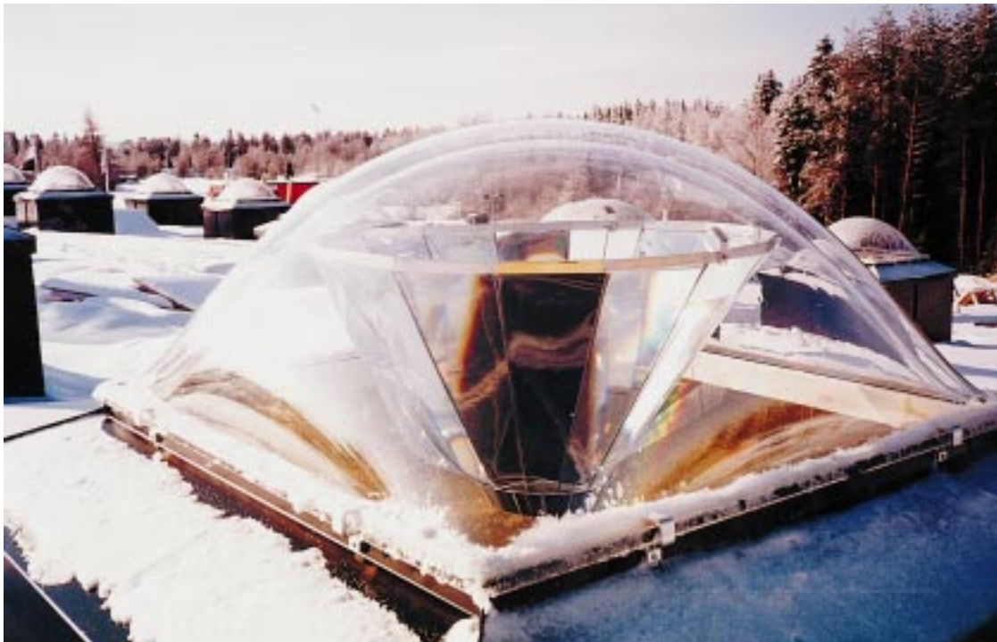
The daylight system showing the two-layer domes with the prismatic cone installed on a roof
